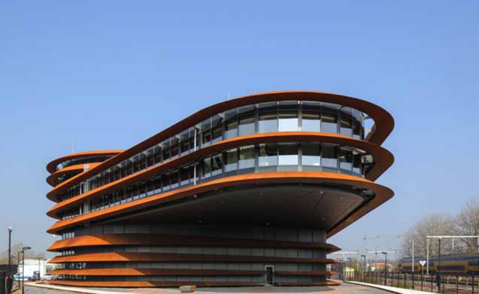
TRAIN CONTROL CENTRE Utrecht, The Netherlands | 2015 by de Jong Gortemaker Algra architects and engineers Photographer: Christian Richters.
