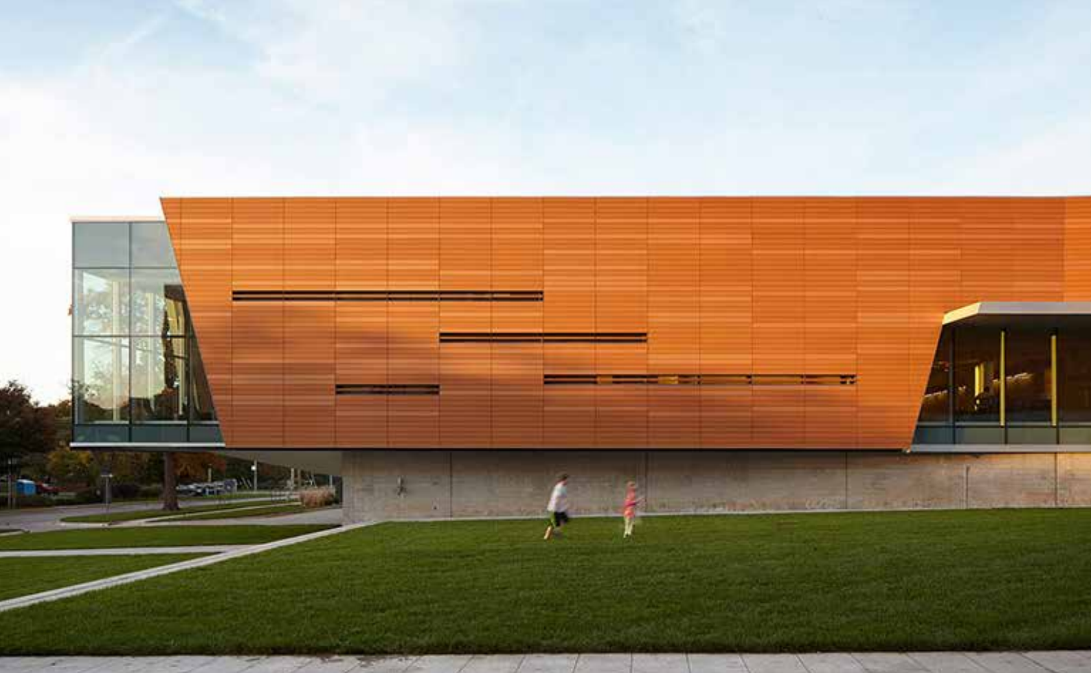
LAWRENCE PUBLIC LIBRARY Lawrence, Kansas | 2014 by Gould Evans Photographer: Tim Griffith Architectural Photographer / Michael Sinclair
