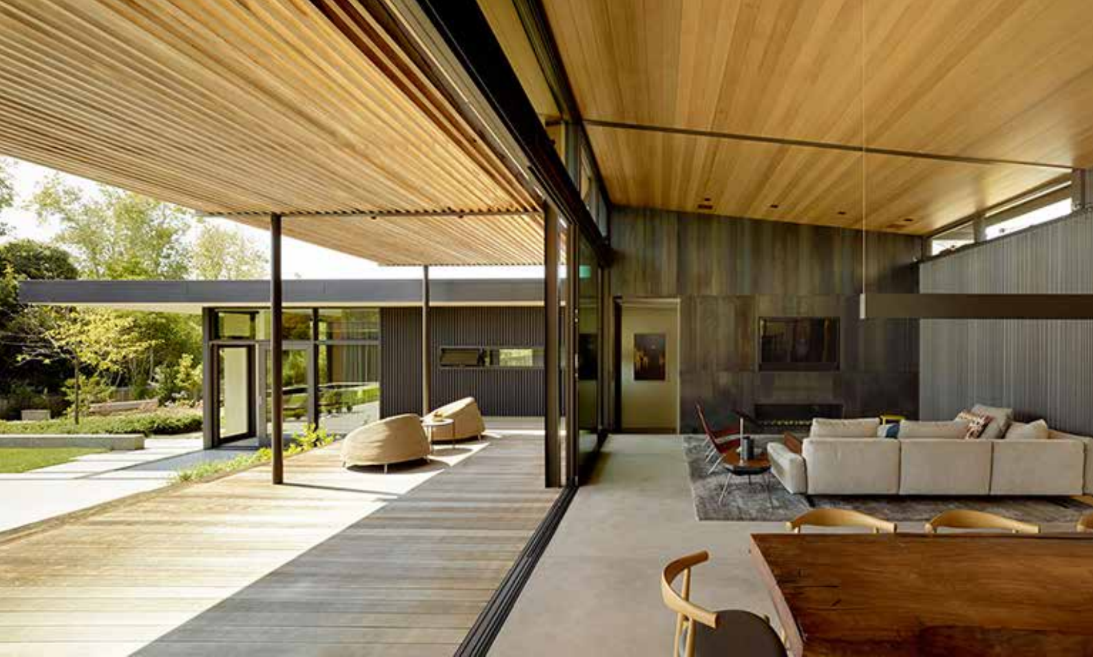
MILL VALLEY COURTYARD RESIDENCE Mill Valley, California | 2014 by Aidlin Darling Design Photographer: Matthew Millman
